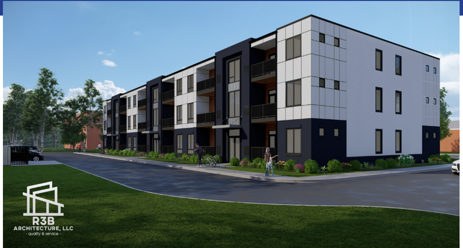
Apartments by Volumod in process at 16th St. & MLK Jr St. in Indianapolis
